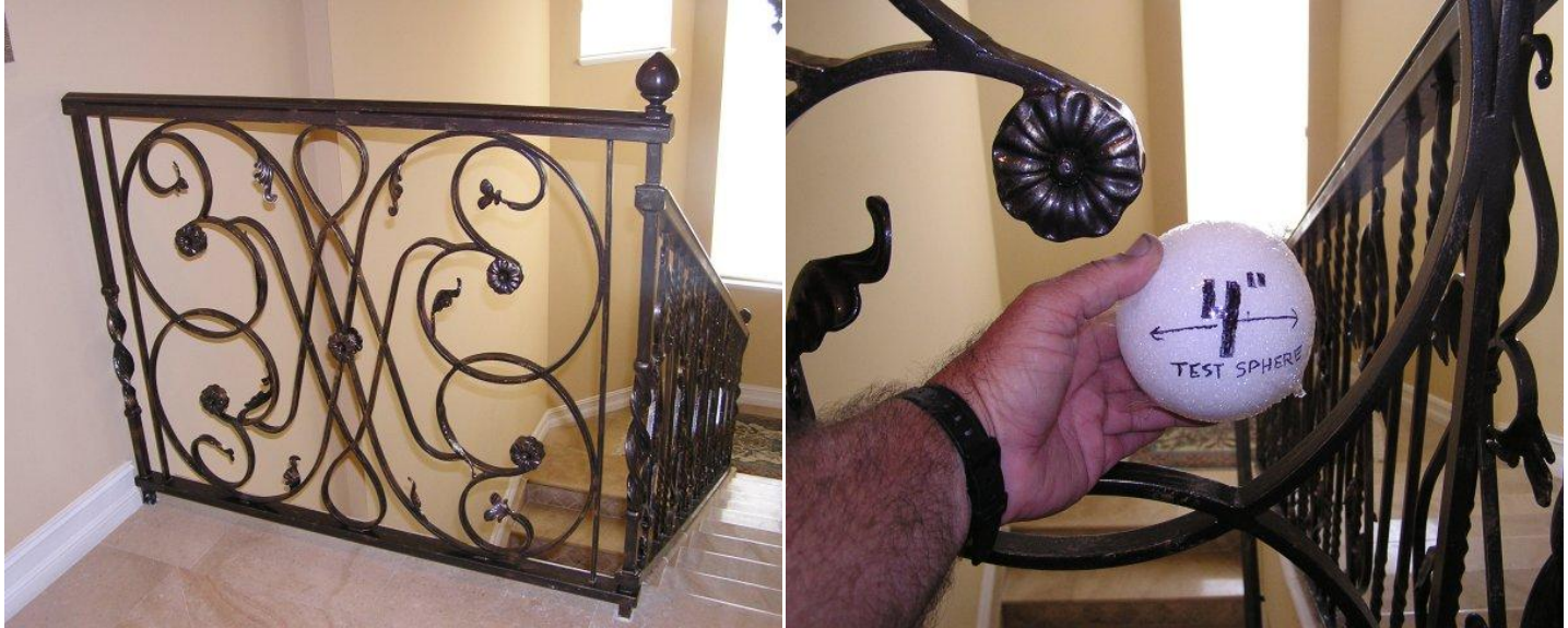
This is showing a 4 inch test sphere in guard infill openings which far exceeds the allowed opening size of "shall not have openings which allow passage of a sphere 4 inches (102 mm) in diameter".
