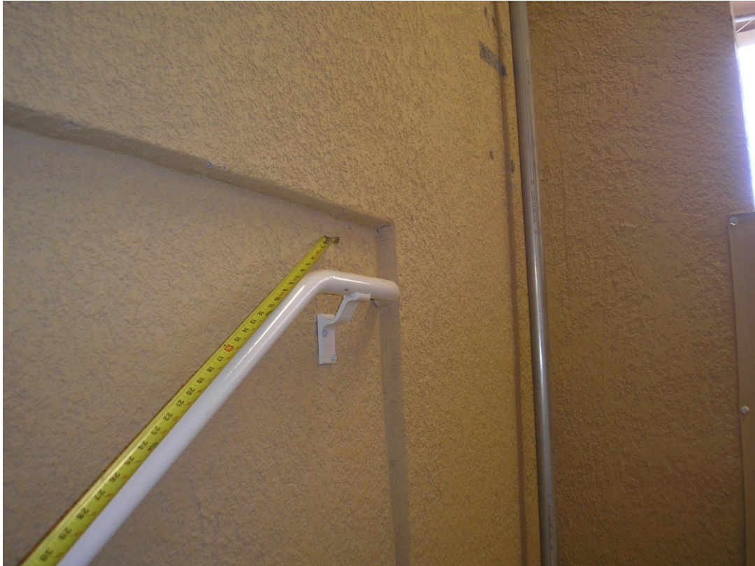
If the stairway is not wide enough ... find a way to make it wider ... recess the handrail.
